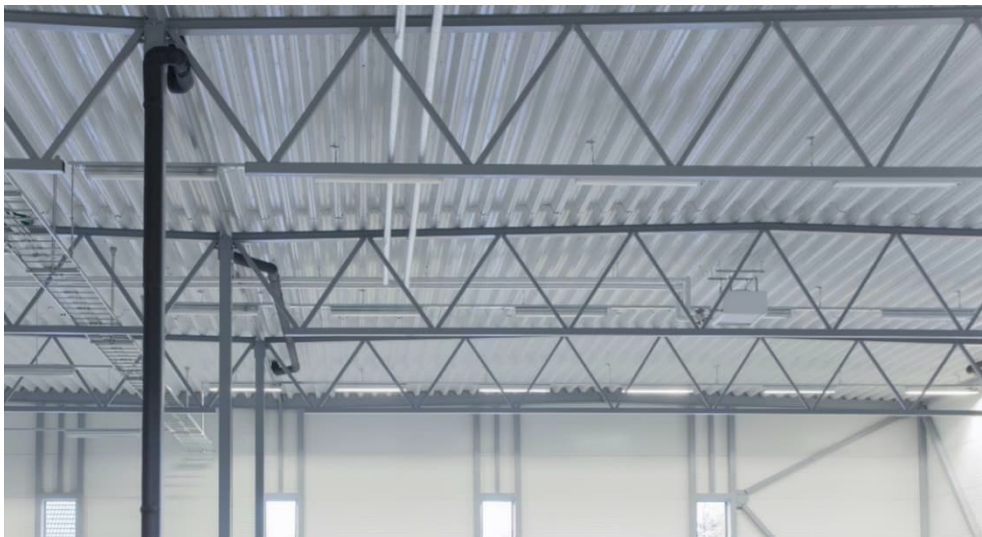
Fig. 4.23 Example of roof system with deep decking [31]
