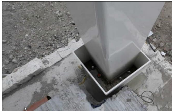
Fig. 4.9 Example of accessible base connection [30]
