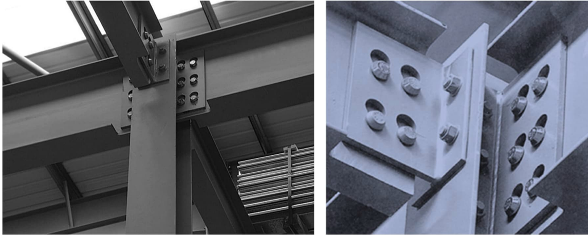
Fig. 4.16 Quicon connections [34]
