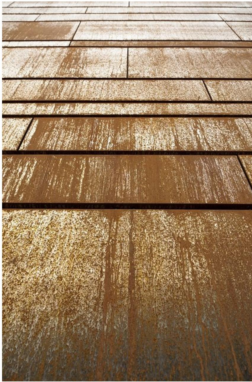
Despite its patina appearance, the steel is resistant to all types of weather conditions. The addition of copper, chrome, nickels or phosphorous gives the steel a self-protecting, oxidized surface. This means that roof and facade cladding are practically maintenance-free, eliminating the cost of painting.
