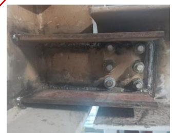
two flanges added for gusset plate
